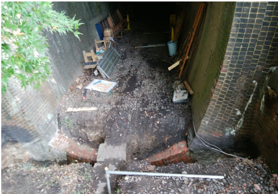
Photo 2 Invert excavation scene
